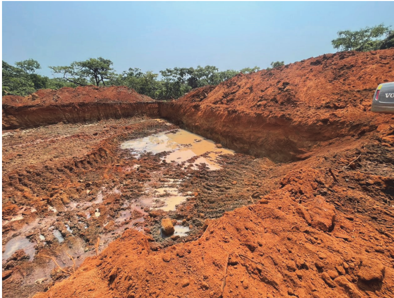
Picture: Preparing to extract a kimberlite sample at L188 following overburden stripping
