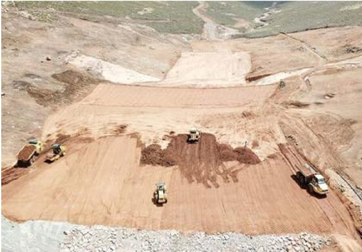
Figure 4: Construction of the wall for the 500,000m<sup>3</sup> water dam at Mothae during the Quarter
