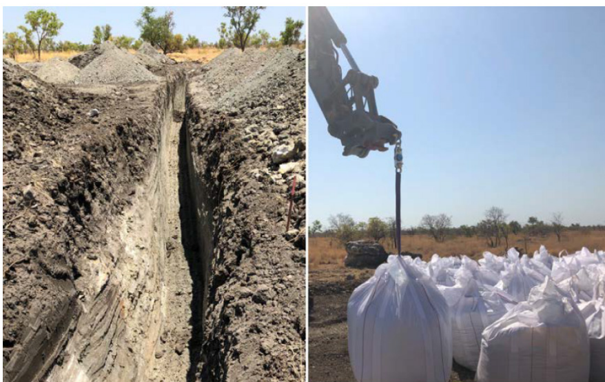
Trenching and bagging of lamproite bulk sample from Little Spring Creek
