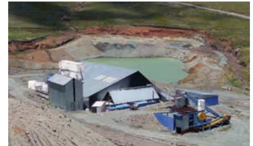
View of the existing processing plant at Mothae.
